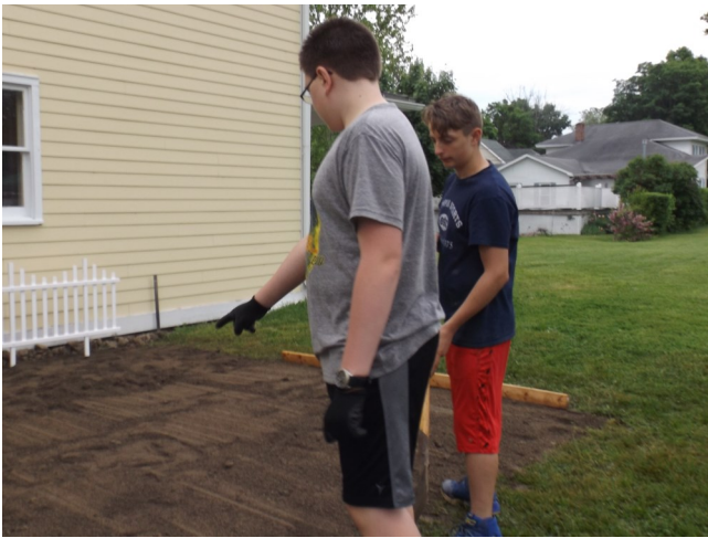
Noah and Robert consult on work being done.
